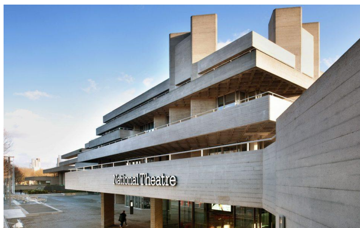
National Theatre, Southbank, London SE1
